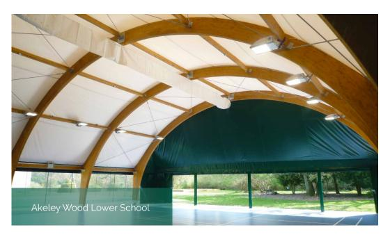
The material - a PVC-coated polyester fabric is self-extinguishing and resistant to abrasions, UV damage and designed to last for more than 20 years.
