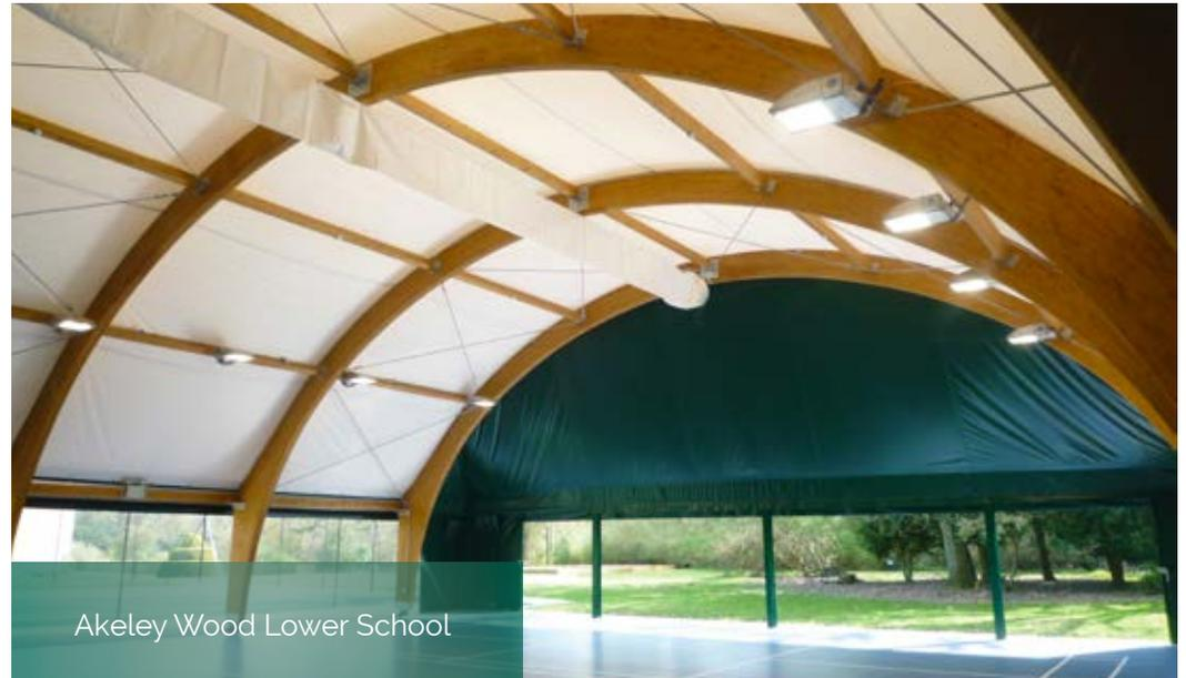
The material - a PVC-coated polyester fabric is self-extinguishing and resistant to abrasions, UV damage and designed to last for more than 20 years.
